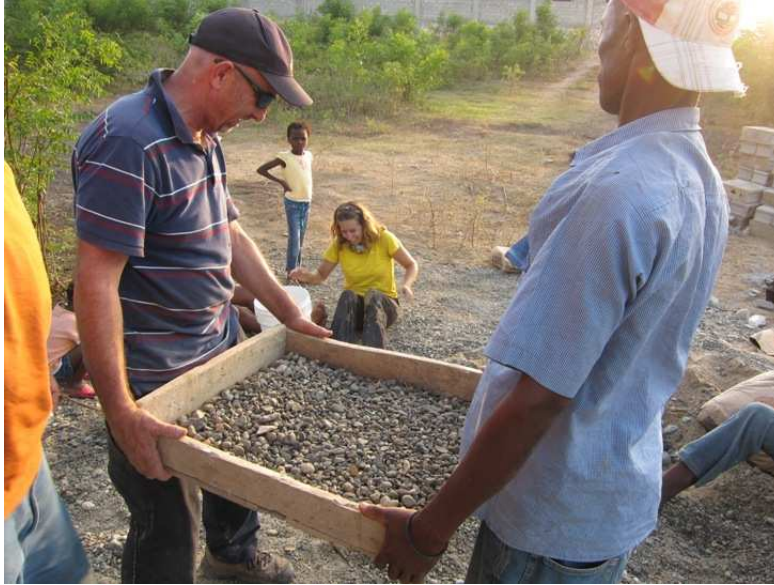
Picture 17: Steve is sifting the rocks to get the right size to use as filter stone
