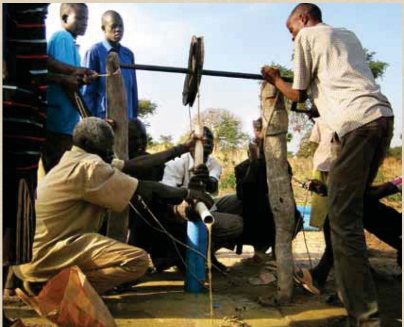
Top: Terry and Hydromissions’ Jen Lorch drill a 50-foot bore hole in Dushanbe with low-tech equipment. Bottom: Muddy at first, water begins to pour from the well Terry and the villagers dug in Ngapacot. Locally available materials make for a crude rope pump that can be maintained easily and provided clean water to the village for the first time.
